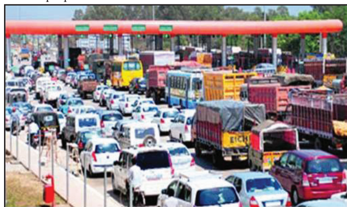
Fig. 1: Existing Inconvenient Toll Tax Collection Method
